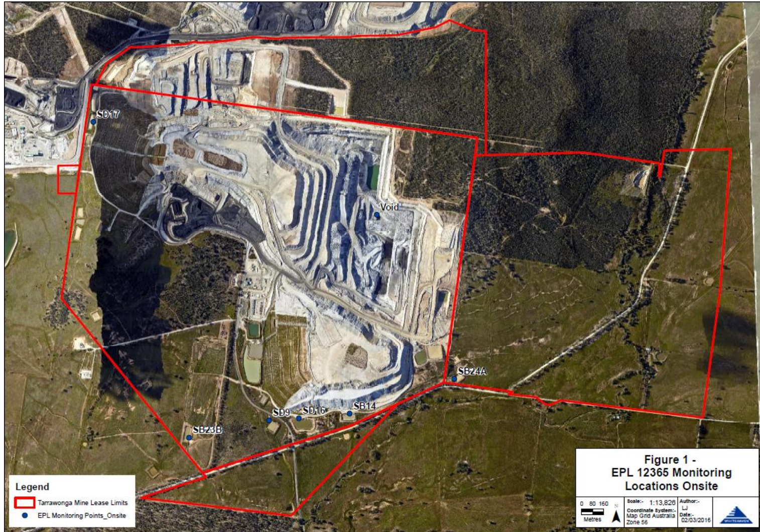
Figure 1 – EPL 12365 Onsite Monitoring Locations
